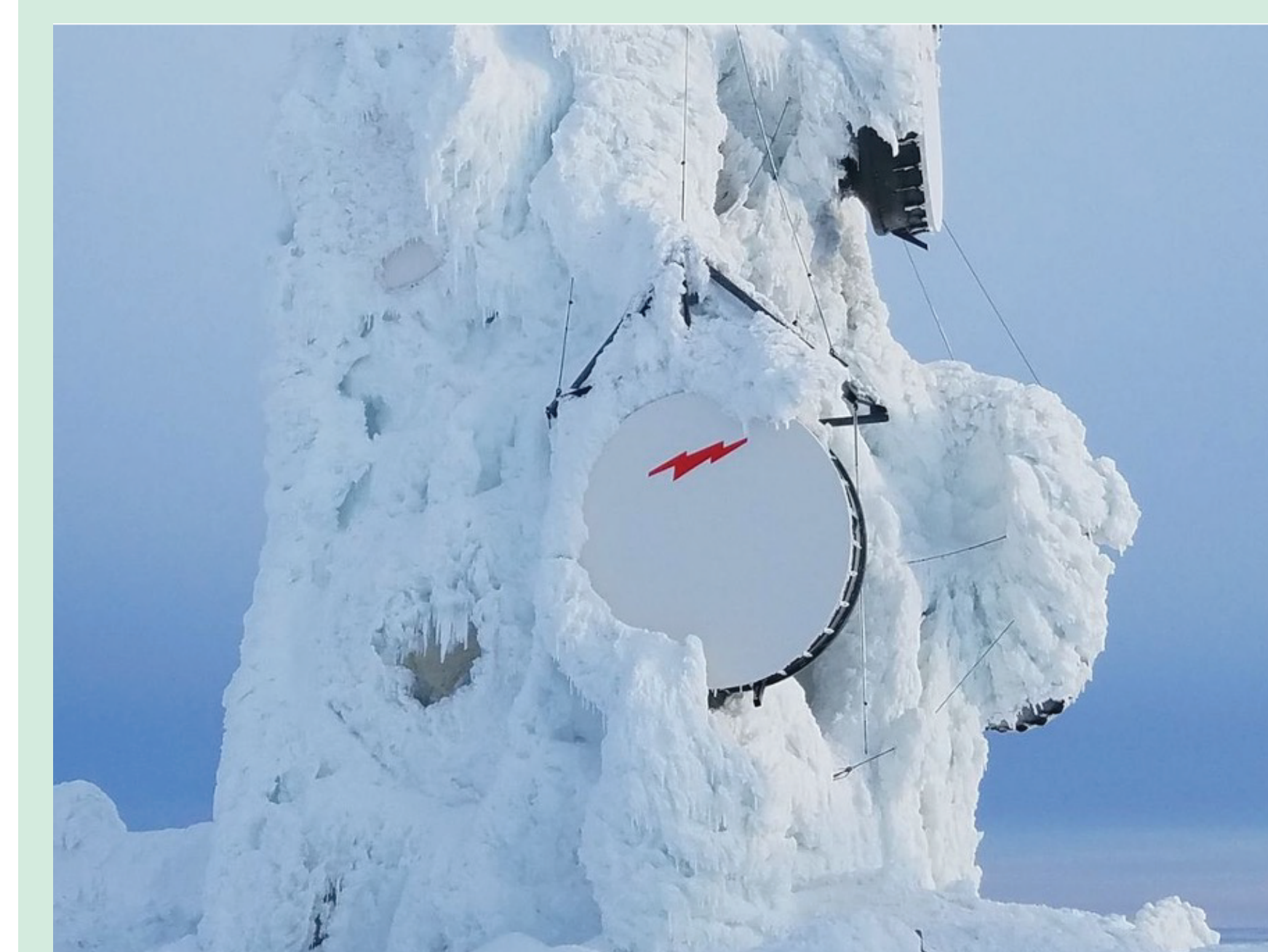
After a rain-on-snow event this cellular tower turned into an ice-crust snow tower, disrupting cellular service in western Alaska in 2018. Credit: www.adn.com
